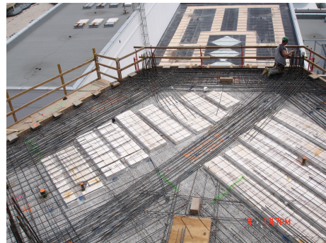
Figure 5: Filigree Construction Photo
